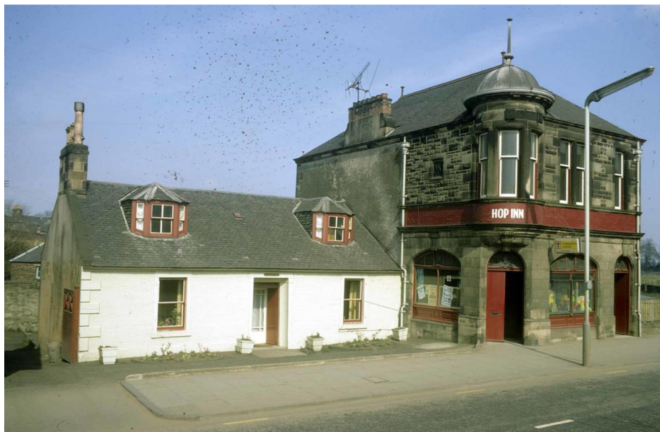
Original Blue Bell Inn, by then a house named Jessmar Cottage, with 2-storey expansion, laterally known as the Hop Inn. Falkirk Archives.
